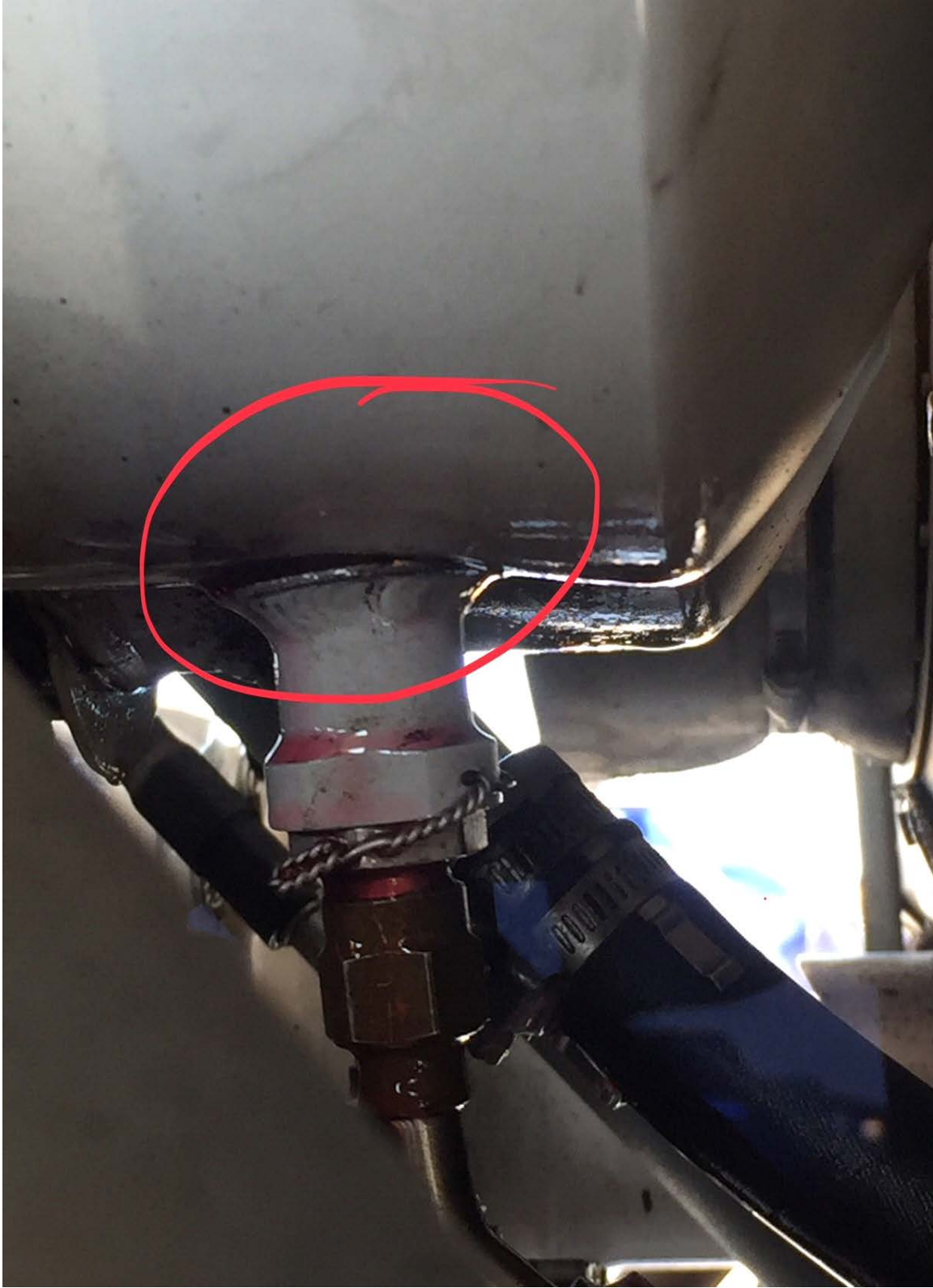
Cracked Hydraulic reservoir suction line base
