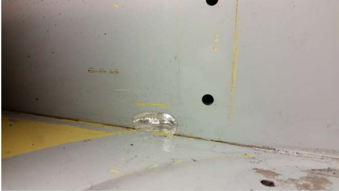
Figure 3 – Final blend-out of corrosion damage
